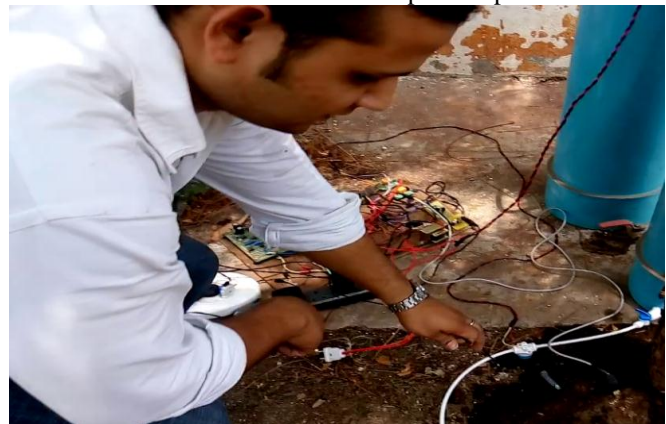
Figure 4.2: Testing valves operation
